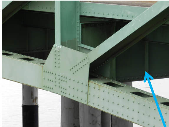
Beam supporting the roadway deck
